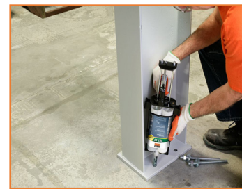
SET & SETXP can be dispensed with a caulking tool.
